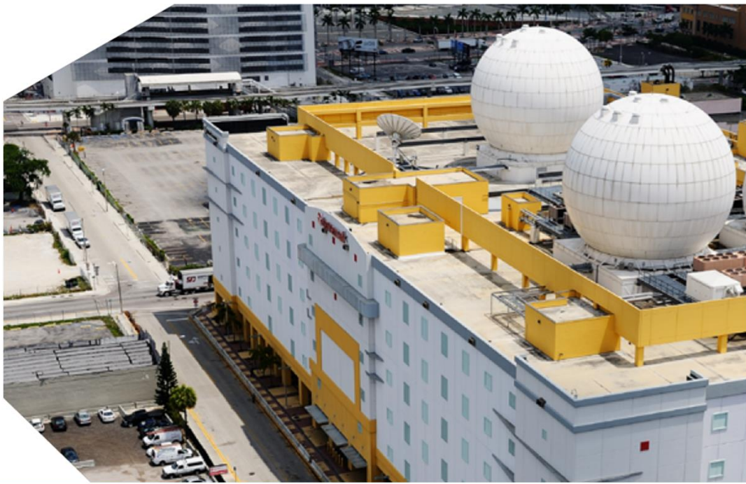
GIGAS. TERREMARK's DATACENTER (MIAMI)
